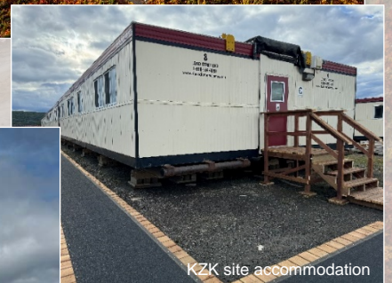
KZK site accommodation
